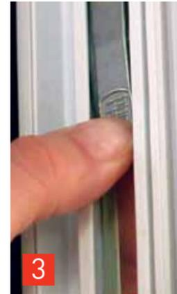
3 Once the safety catch is released the window can be completely rotated
